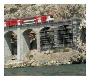
The Works fulfilled can be broken down into three clearly different operations. The first consists of the construction of a service way which is built on the side of the bridge in cantilever. The second is the general operations of cleaning and structural rehabilitation, consisting in high-pressure cleaning of the face and
